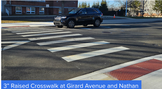
3" Raised Crosswalk at Girard Avenue and Nathan Hale School, New Haven, CT, installed 2022.
