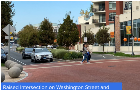
Raised Intersection on Washington Street and Commerce Park, Stamford, CT, installed 2011.
