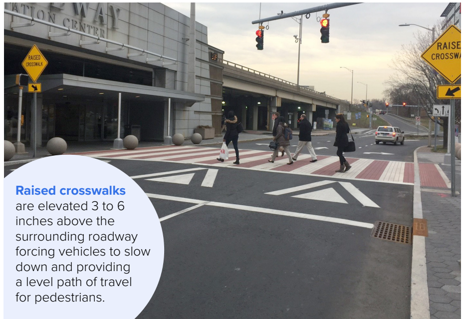
Raised crosswalk on North State Street, Stamford, CT
