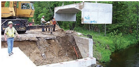
Photos courtesy of FHWA
