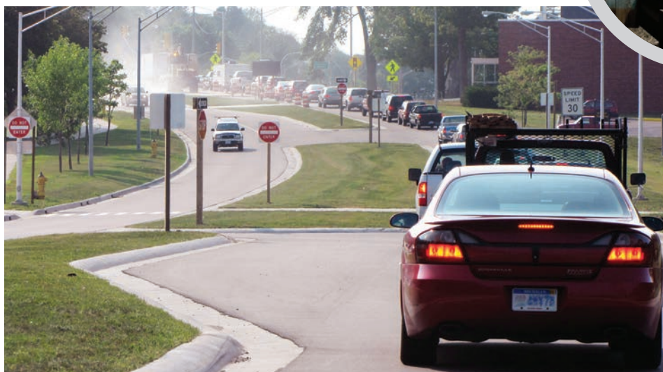
Dedicated turn lanes, pedestrian refuge areas, adequate signage, and wide separation between traffic lanes all contribute to the safety of a road. The new Highway Safety Manual provides guidance for determining the best treatments to address safety concerns.
