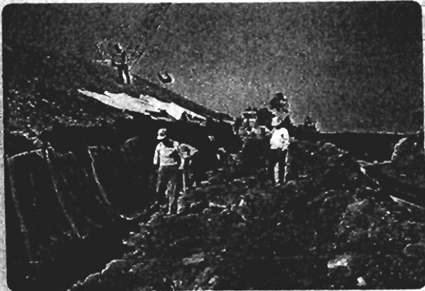
3. Prefabricated Underdrain Being Placed
