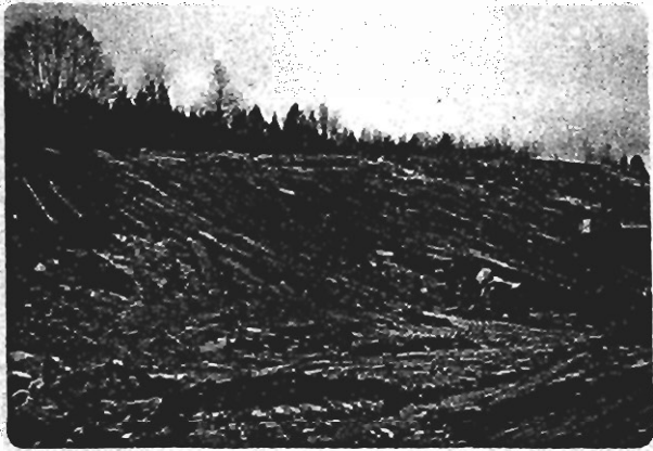
1. Slope April 1971, Note Wet Areas & Manholes
