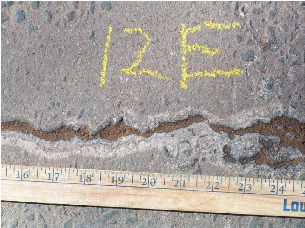
**Figure 4: Failure of cold material (cohesion/adhesion)**
