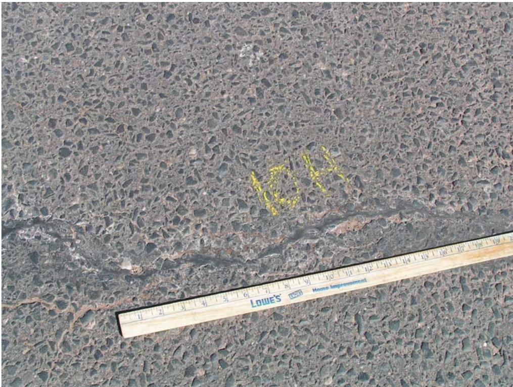
**Figure 2: Failure of hot material (cohesion/adhesion)**
