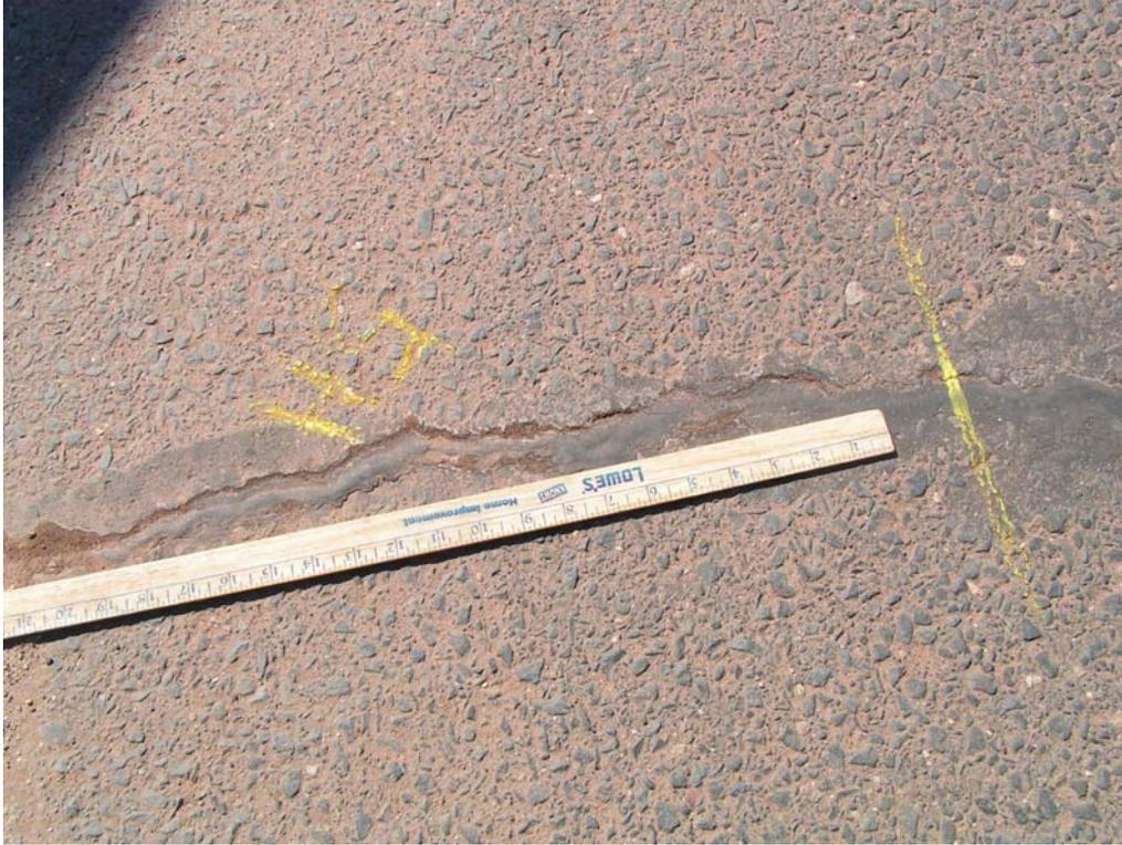
**Figure 1: Failure of hot material (cohesion/adhesion)**
