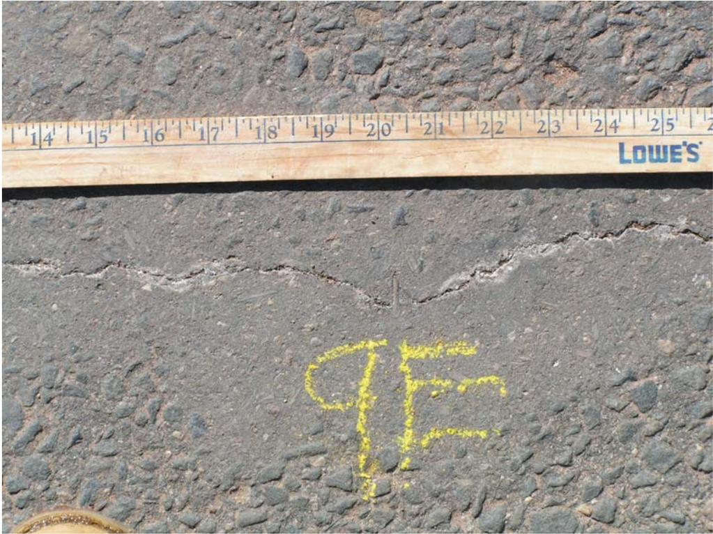
**Figure 3: Failure of cold material (cohesion/adhesion)**
